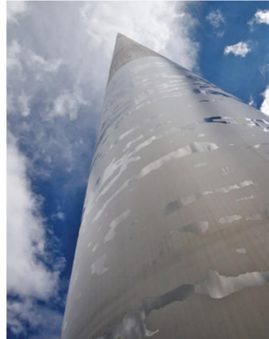
The Dublin Spire – a stunning example of our surface texturing technique showing the versatility of controlled shot peening
