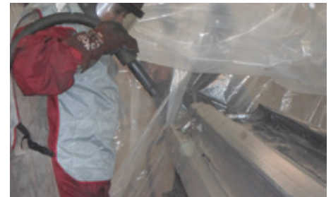
Shot peening technician working on a localized area of concern
